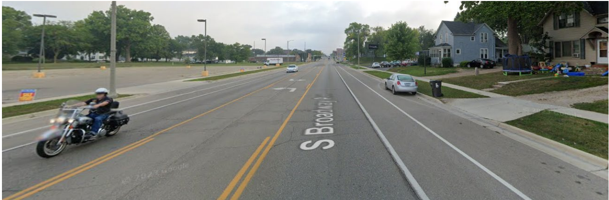
Figure 25. Photo of Highway 65 / South Broadway in Albert Lea, MN before (top) and after (bottom) road redesign.
